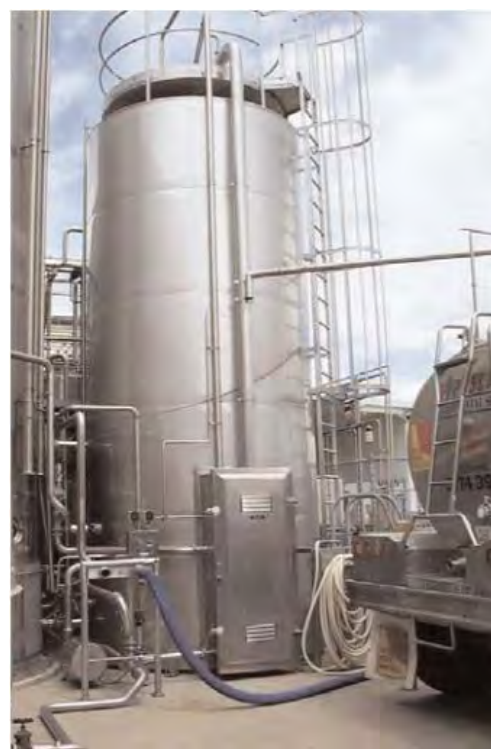
A dedicated storage tank for stockfeed. Dairy processing wastes such as separator de-sludge, whey and product returns are a good source of protein and fat and are often used as animal feed.
