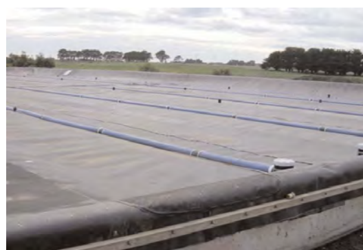
Anaerobic digestion of food-processing wastewater produces biogas that can supplement energy requirements.
