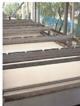
Primary treatment systems such as induced air flotation (IAF) are commonly used in the dairy processing industry to remove fats and suspended solids.
